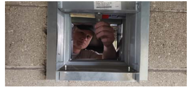
MAINTENANCE FIRE DAMPER
